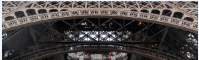
The Eiffel Tower is a classic example of lattice structure design.
